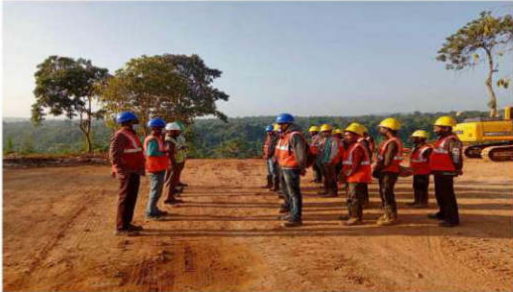
Fig -4. Daily Prestart Briefing before start of work.
