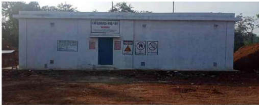
Fig -3. Display of Safety Warning and Cautionary Signe board for Explosive Magazine.
