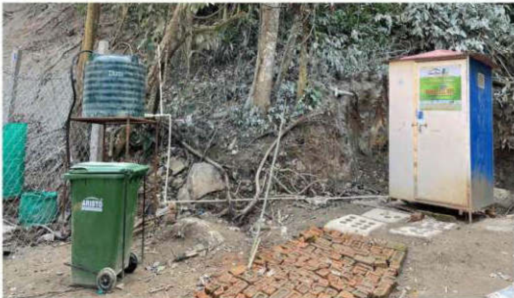
Fig: Portable toilet installed at Adit to HRT location.
