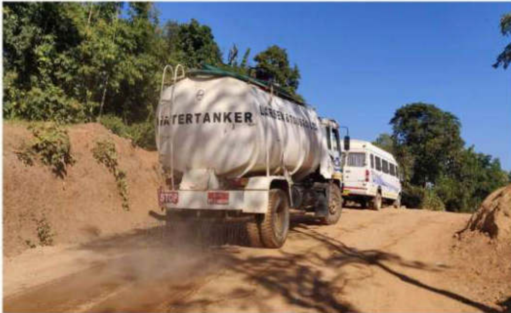
Fig: Water sprinkling on road to reduce dust pollution.
