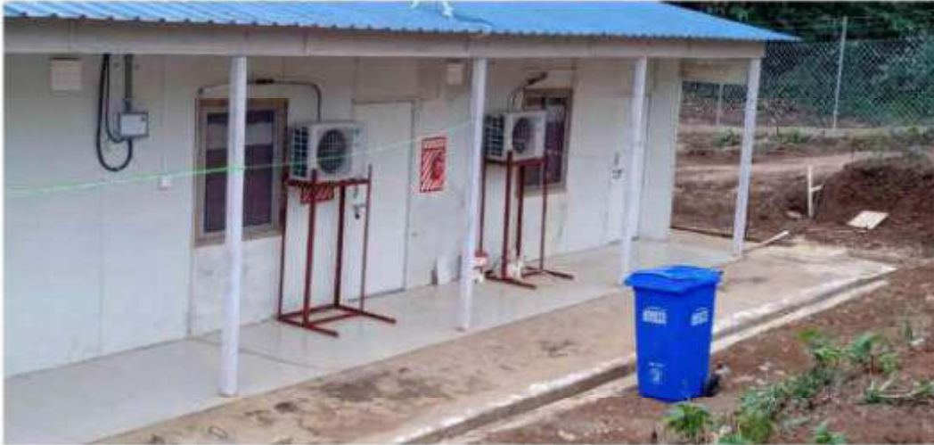
Fig -15. Fire Extinguisher provided for all PMC Blocks
