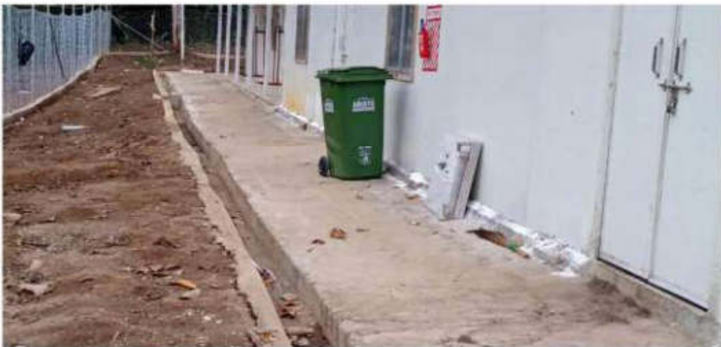
Fig -16. Fire Extinguisher provided for all PMC Blocks
