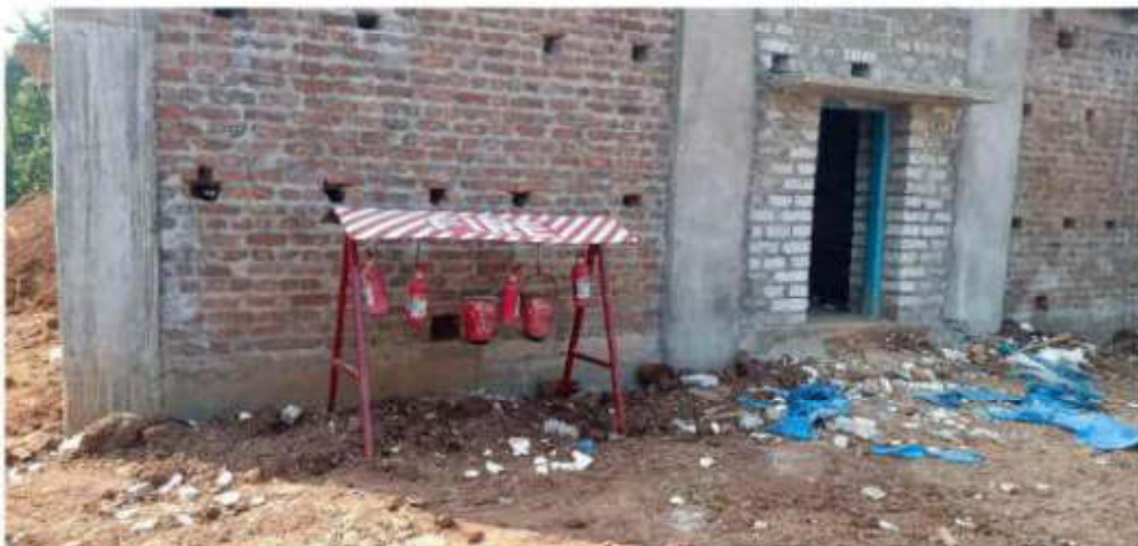
Fig -18. Fire Stand at Explosive Magazine
