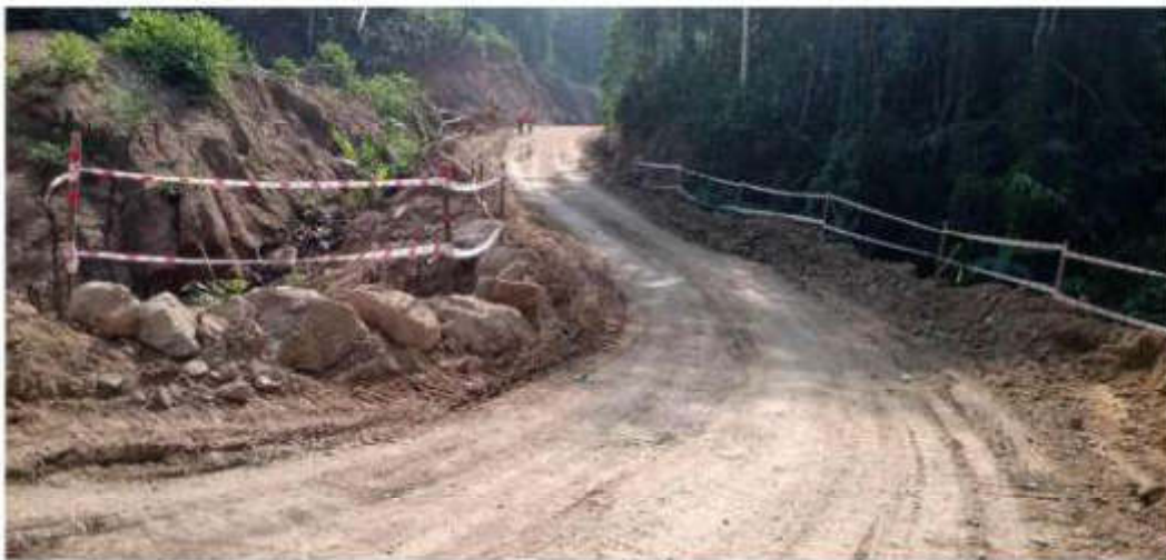
Fig -9. Temporary edge protection by Cautionary tap
