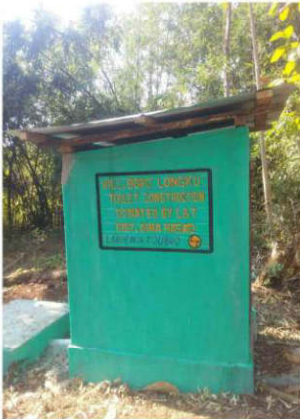
Fig: Community toilet constructed by L&T for local villagers.
