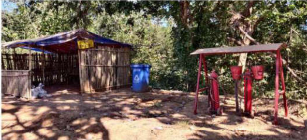
Fig -19. Fire Stand at Surge Shaft
