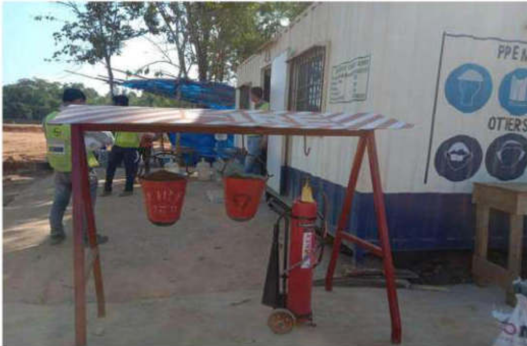
Fig -17. Fire Stand at Valve house Office
