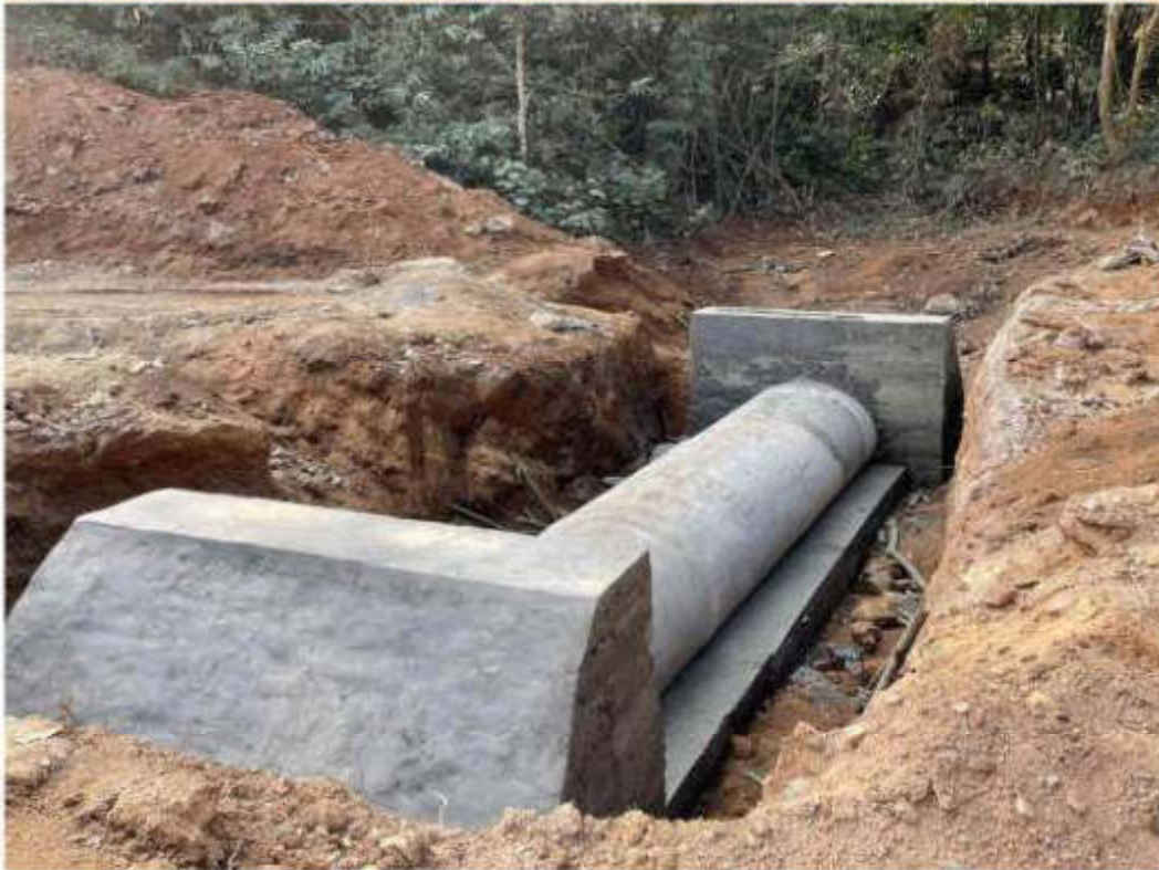
Fig: Culvert & drain work inprogress.
