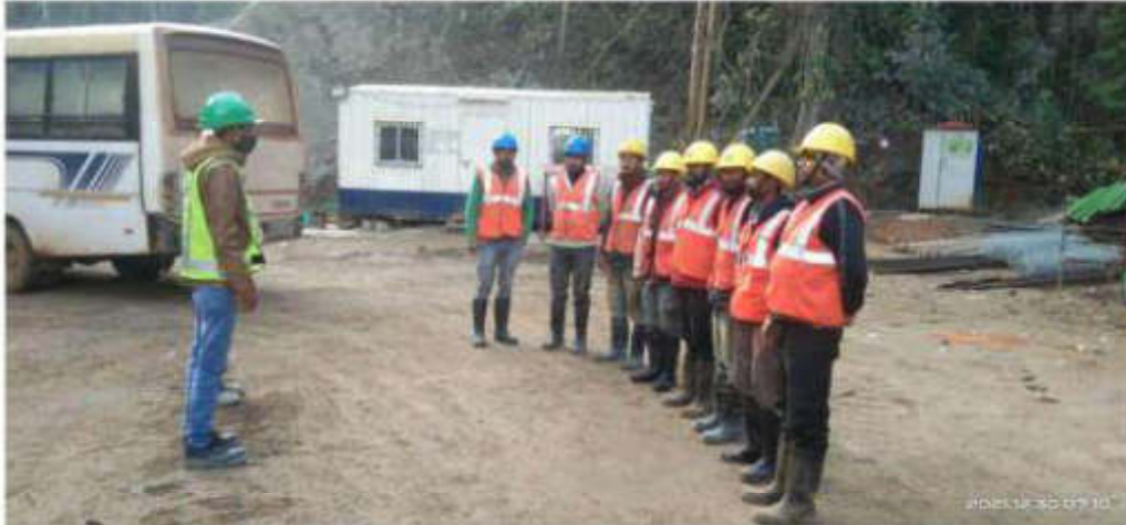
Fig -2. Daily Prestart Briefing before start of work.
