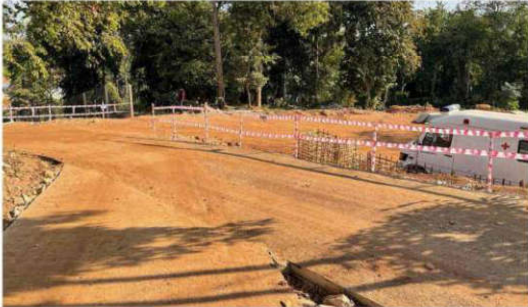
Fig -8. Barricading by Cautionary Tape
