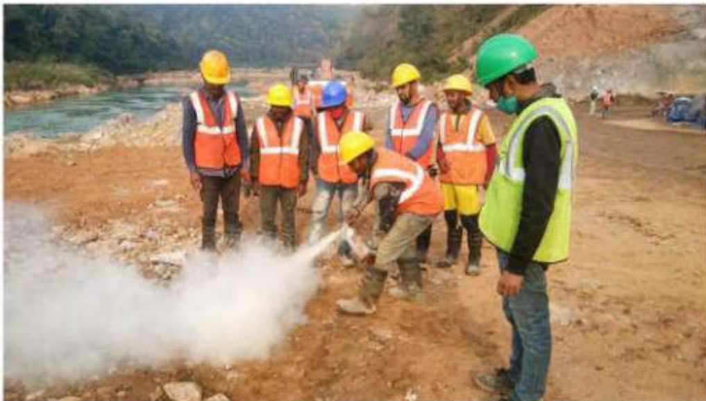
Fig -3. Fire Safety
