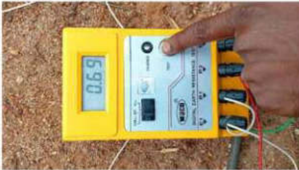
Fig -11. Periodical Earthing Resistance Monitoring
