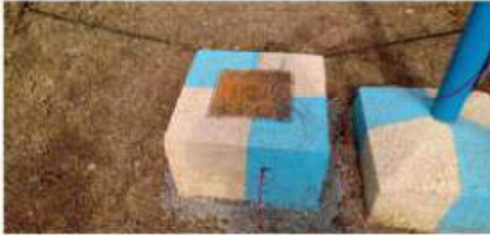
Fig -10. Slanted Earth Pit for Electrical equipment
