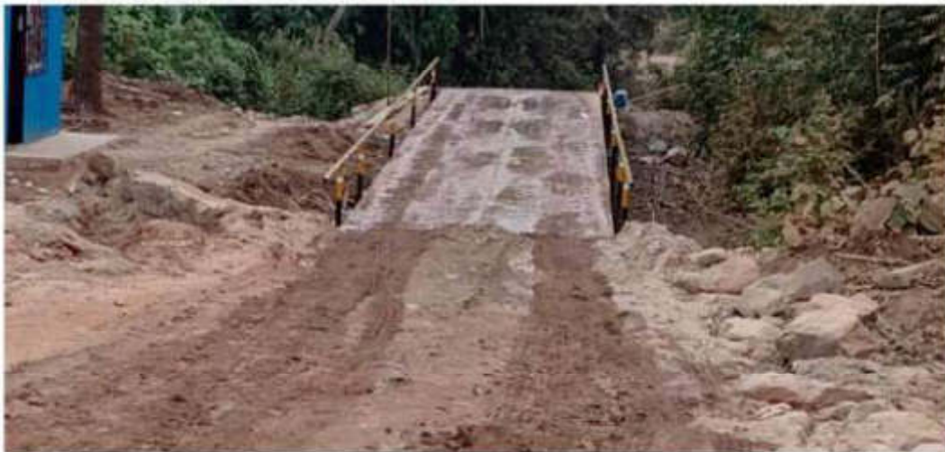
Fig -7. Edge protection for weighbridge
